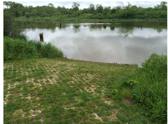
Stabilized natural surface access using Turfstone at Lewis and Clark National Historical Park, Washington. Photo Credit: Brian Rushing
