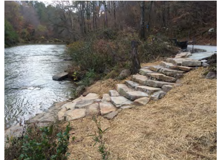
Native stone steps at Grants Mill access that sit within the natural river bank profile. Photo Credit: Brian Rushing
